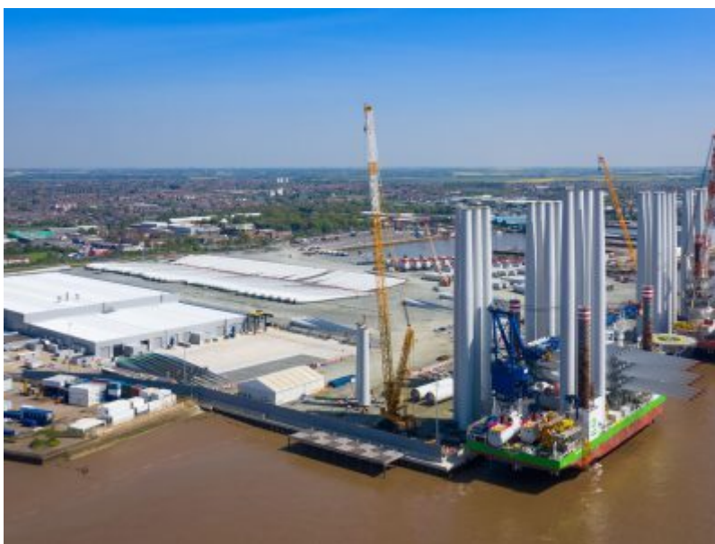
Fig. 2: Green Port Hull, https://greenporthull.co.uk/what-we-do/siemens-gamesa
